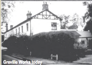
Greville Works today
